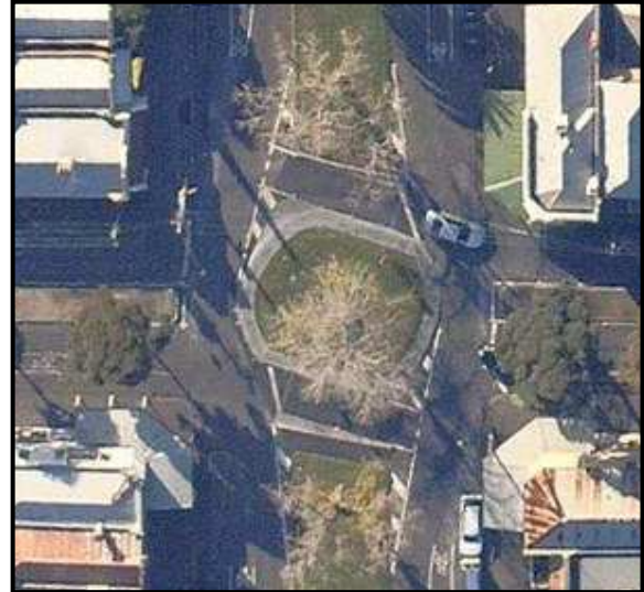
2010: No longer functioning as a roundabout. Stop signs on Pigdon St and within median, and storage in median.
