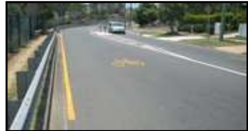
Figure 12: Markings to indicate the desired safe path for cycling within a lane shared with motorists. “Bicycle awareness zone” (BAZ) in Queensland, Australia above; and “sharrows” in Toronto, Canada below.
