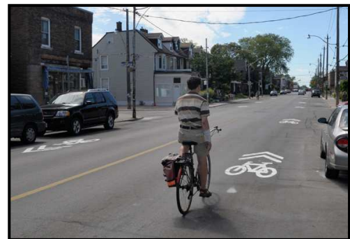
Figure 12: Markings to indicate the desired safe path for cycling within a lane shared with motorists. “Bicycle awareness zone” (BAZ) in Queensland, Australia above; and “sharrows” in Toronto, Canada below.
