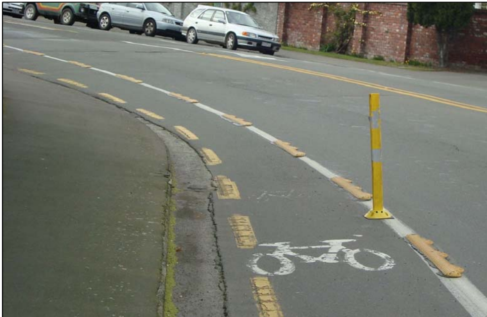
Figure 1: Riley separators and a vertical post installed on Kotare Street cycle lane line
