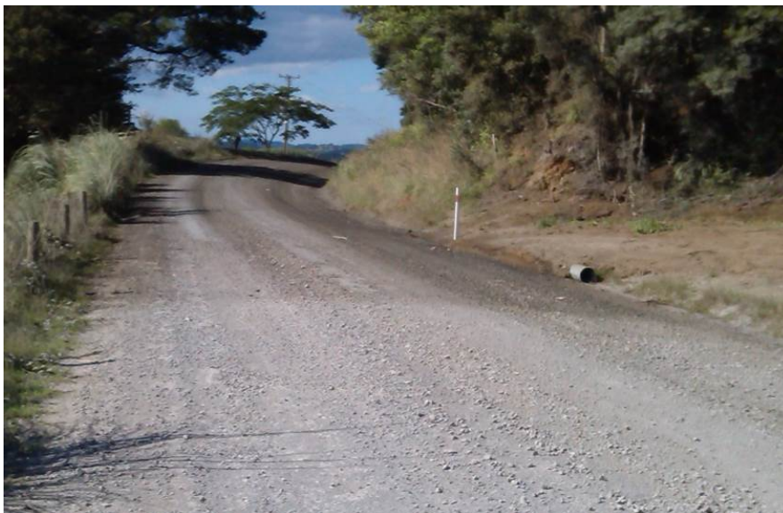
Figure 3.8 Treated (dark upper) and un- treated (light lower) sections of Mataraua Road
