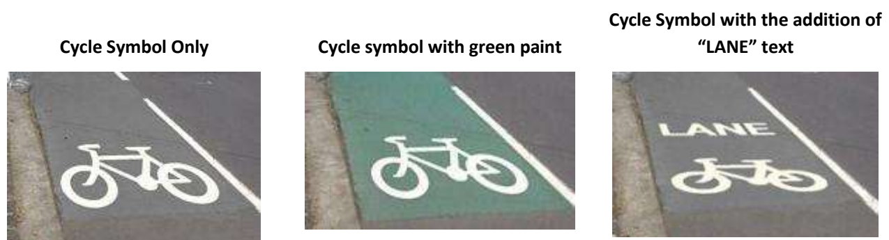
Figure 26: Survey figure of cycle lane markings
