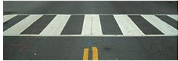
Figure 8. Possible crosswalk marking
