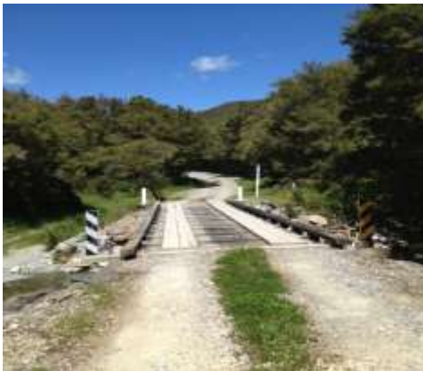
Heaphy track – Eastern access via Aorere Rd
