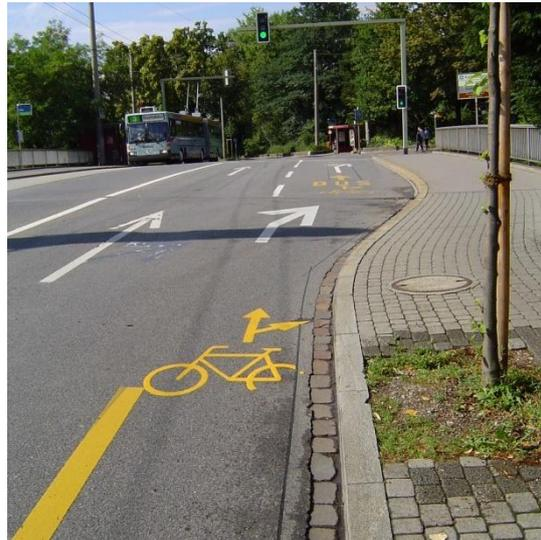
Figure 36: Intersection markings for straight through cyclists in an exclusive turn lane, Switzerland (photo: Axel Wilke)
