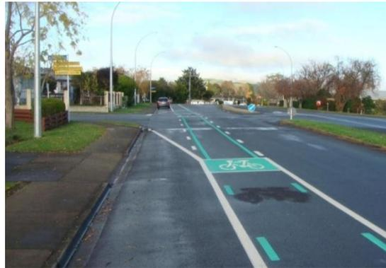
**Figure 41: Dashed and continuous green lines within standard cycle lane at side road**
