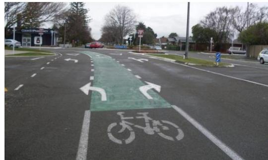
**Figure 23: Roundabout approach cycle lane with arrows to encourage vehicular lane positioning (Palmerston North)**
