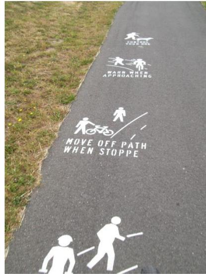
Figure 48: Path user behaviour markings, Railway Path
