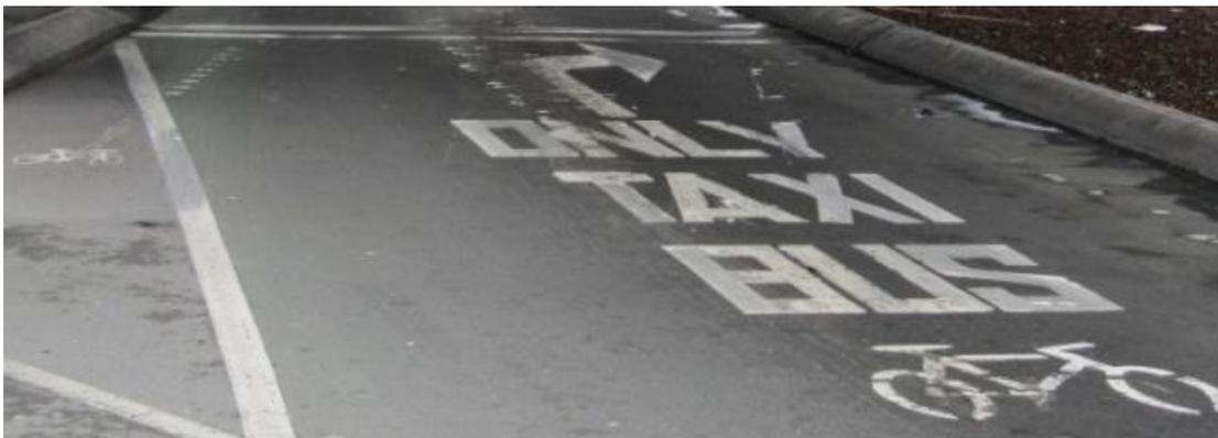
**Figure 3: Special vehicle lane markings**
