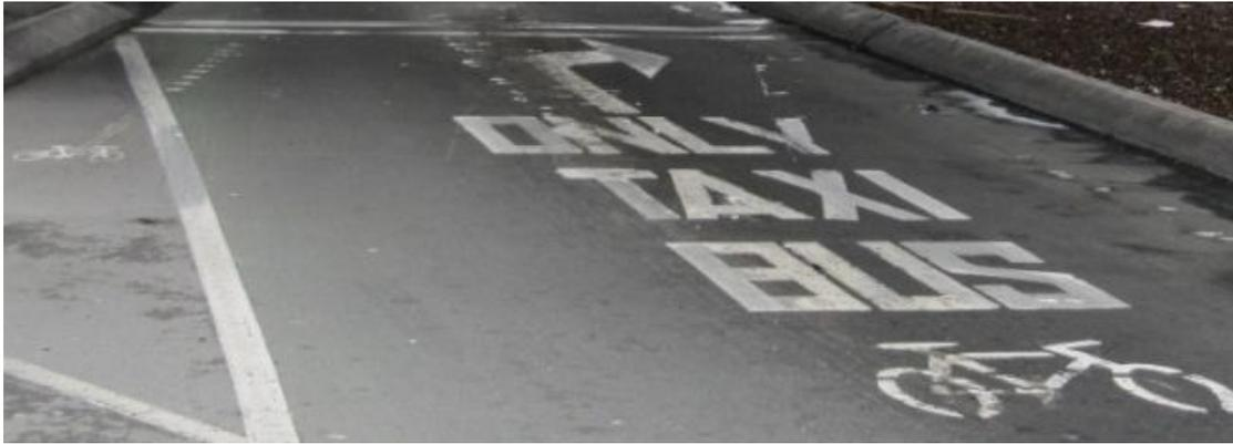
**Figure 3: Special vehicle lane markings**
