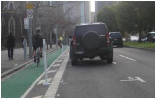
Figure 11: Buffered and flag protected cycle lane between footpath and clearway, Melbourne
