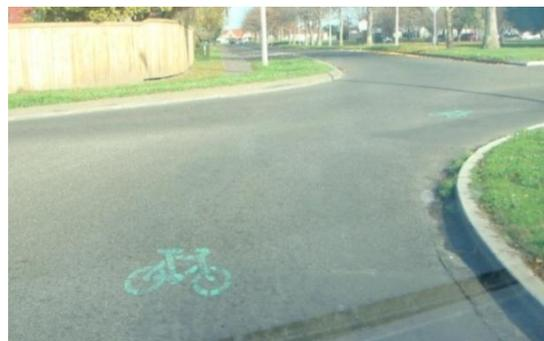
**Figure 24: Green cycle symbol in roundabout (Hastings)**
