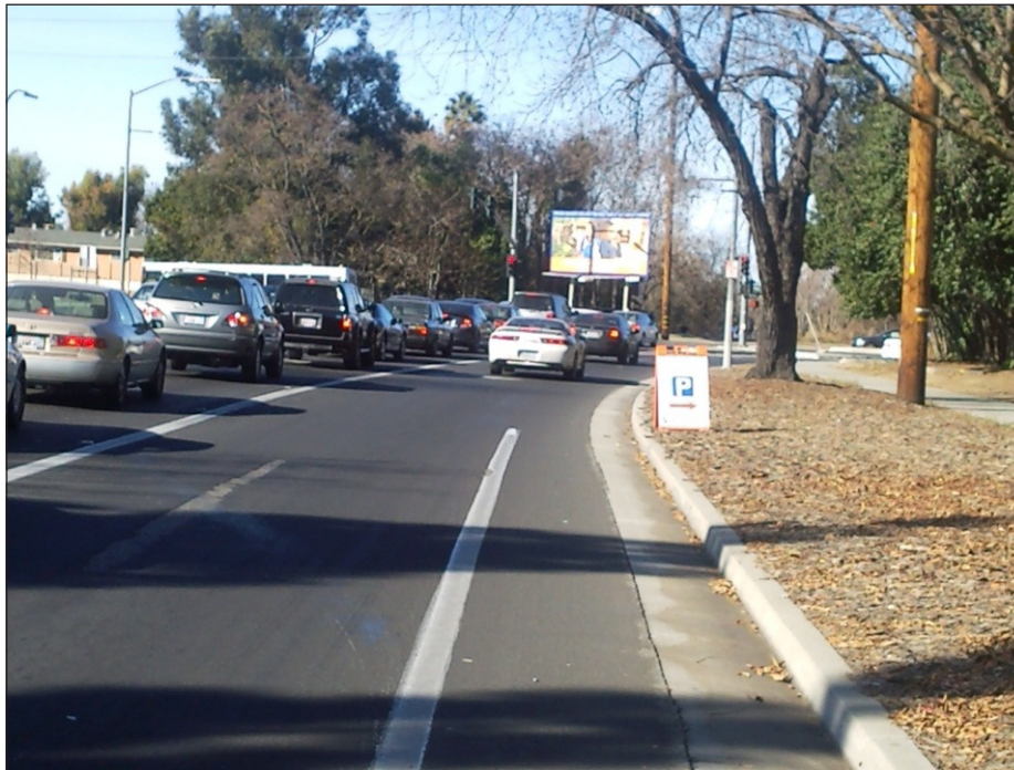
Figure 2. Bike Lane Disappears to Make Space for a Right-turn Lane
