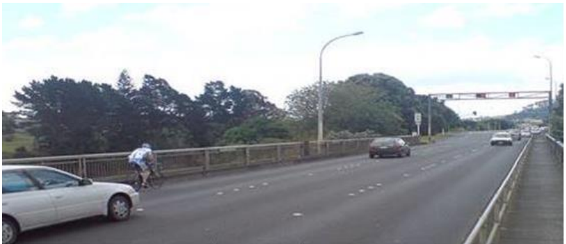
Panmure Bridge, Auckland
