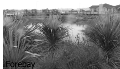
Road stormwater collected in sumps with enviropods and piped to forebay. Roof stormwater directed to roads.
