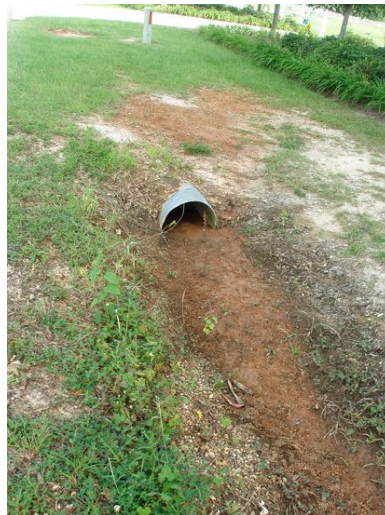
Figure 4: Poorly maintained Swale
