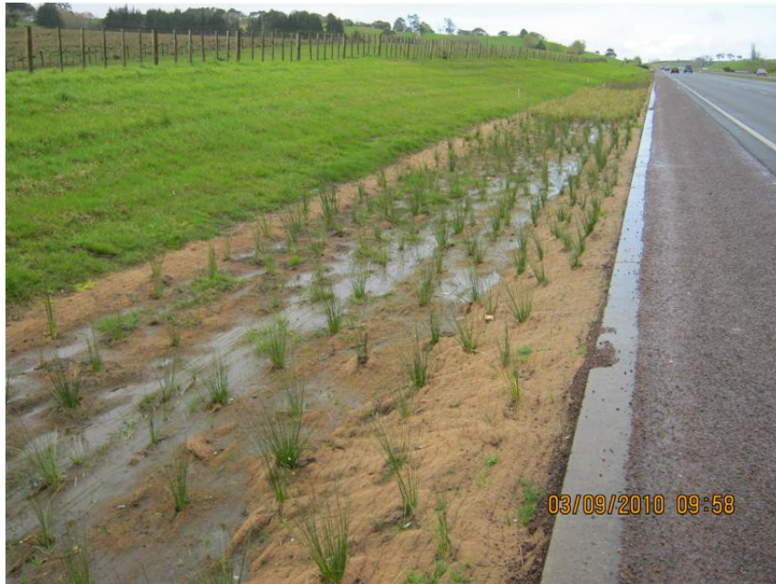
Figure 19: Photo of Silverdale site showing pooling of water
