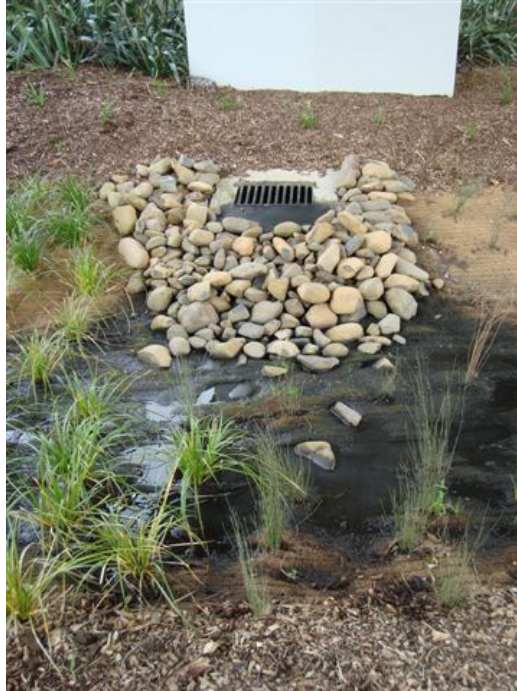
Figure 21: Picture of surcharging catchpit
