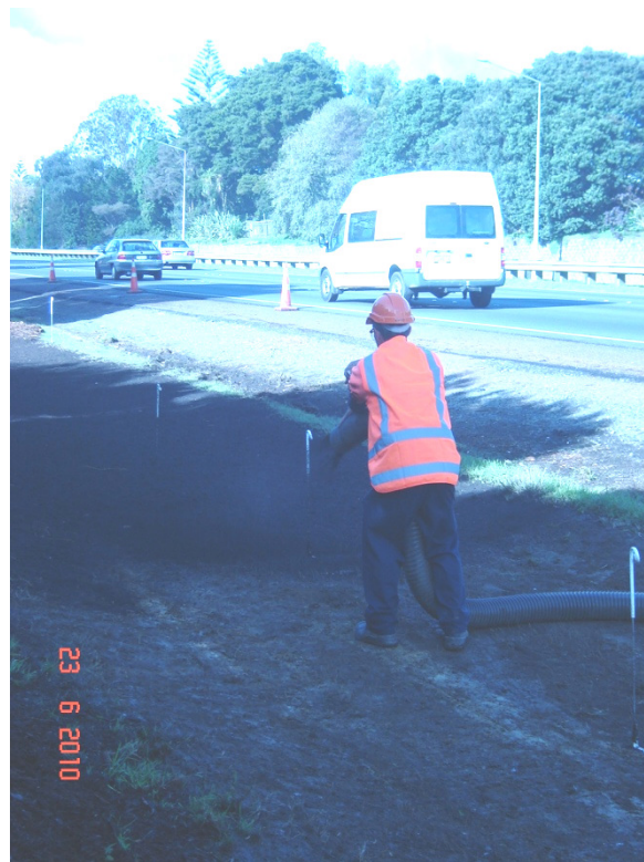
Figure 15: Photo of topsoil application at the Alfriston site
