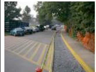
Infiltration trench Source: Washington Cathedral Stormwater Management and Ravine Restoration Programme.
