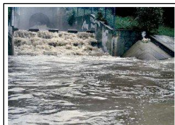
Flash flood through a stormwater outfall
