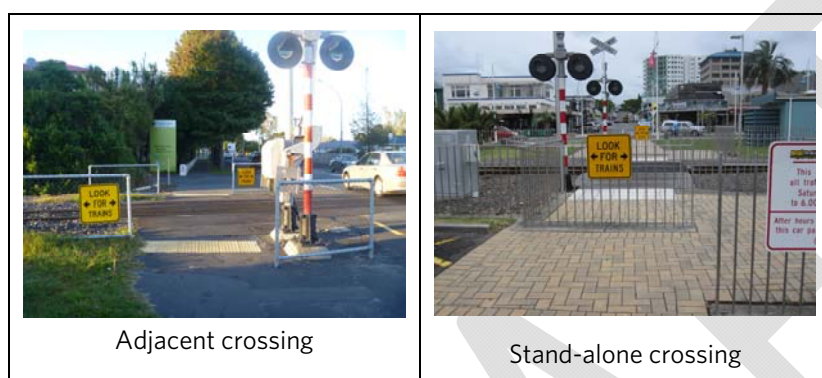
Figure 8 Pedestrian level crossings – photos of two types
