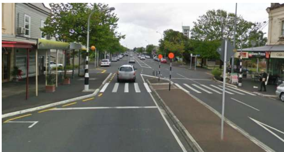
Figure 25: Kerb build out and centre island (Source: Google Streetview)
