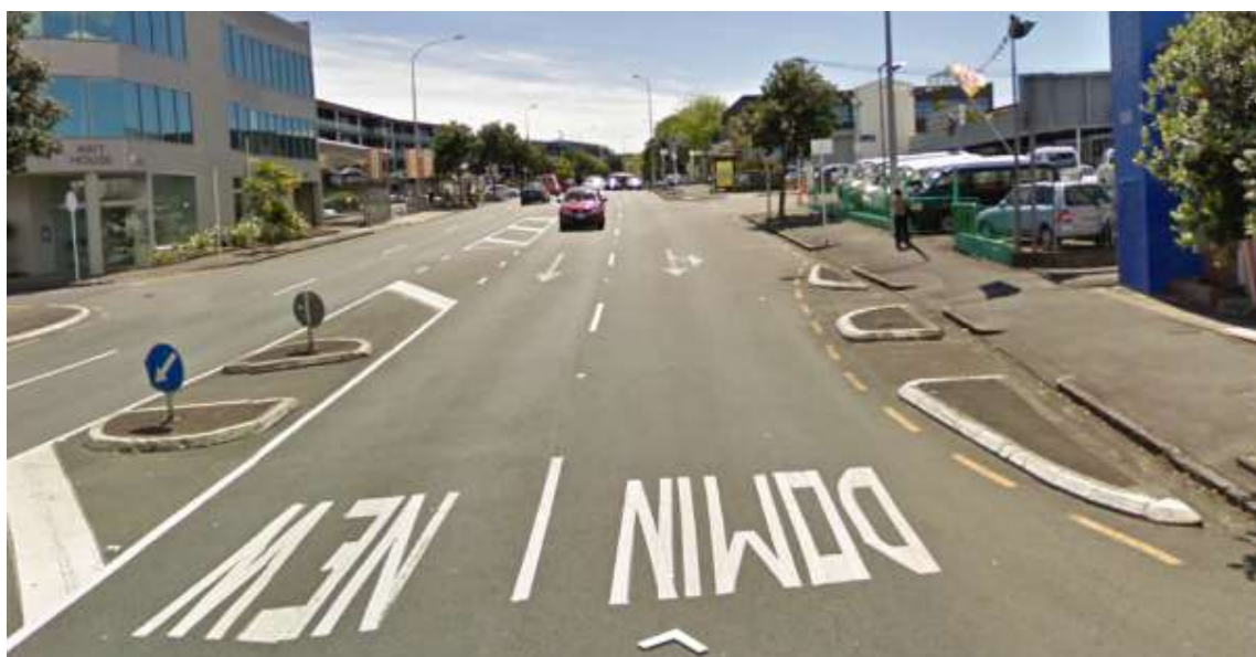
Figure 10: Streetview image of problem area (Source: Google Streetview)
