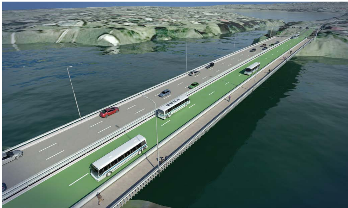
Additional Panmure Bridge – busway and cycle/foot path
