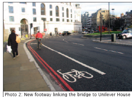
Photo 2: New footway linking the bridge to Unilever House
