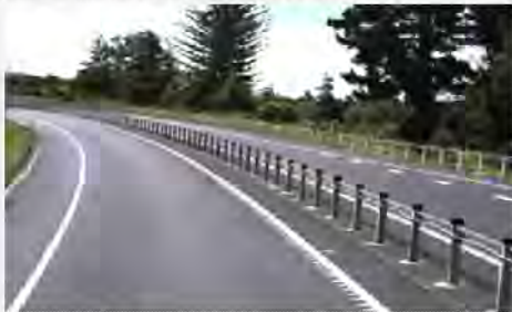
Side and central wire rope barrier, SH1 Rangiriri
