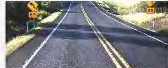
Figure Error No text of specified style in document-1: No-passing centreline with rumble strips
