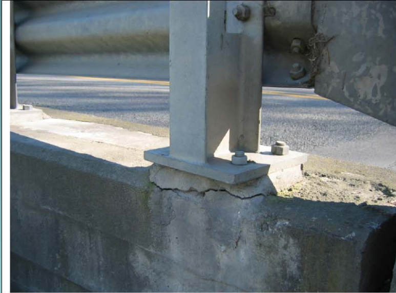
SH1S Ashley River Bridge - Minor Spalling
