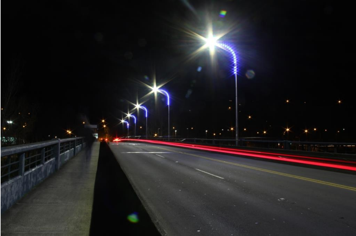
Melling Bridge, Hutt City
