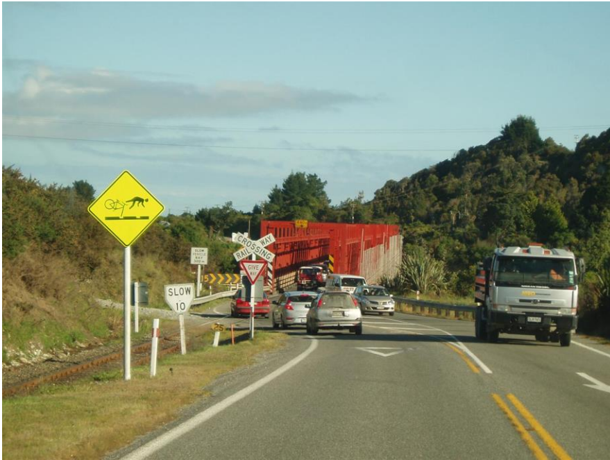
Taramakau Road/Rail Bridge, West Coast
