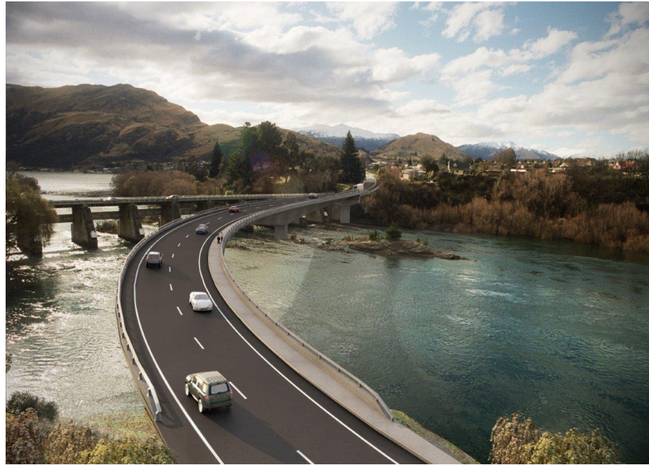
Kawarau Falls Bridge, Otago
