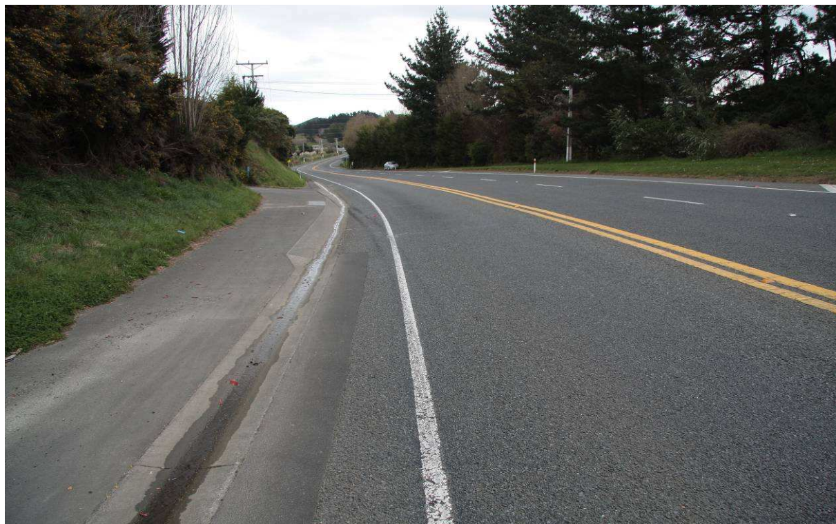
Figure A12 Roadside conditions at Pauatahanui Stream looking north back towards the stream at the base of the hill, again showing the channel carrying water to the stormwater drain pipe.
