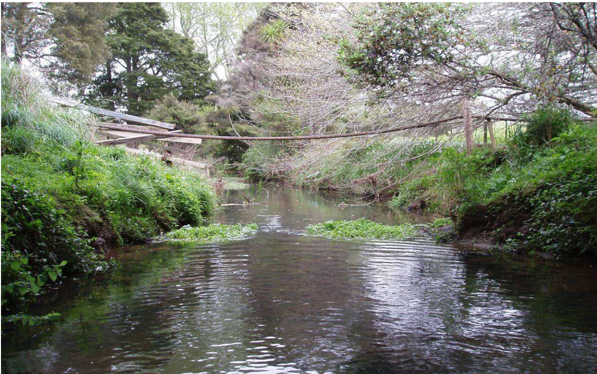
Figure A18 North Branch, Mahurangi River, Site 3 below the road bridge
