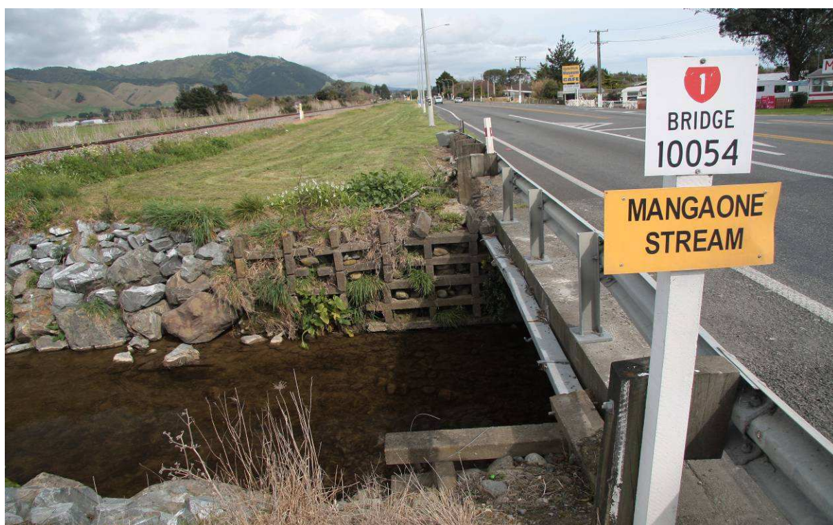
Figure A4 Mangaone Stream looking southward, showing grassy verge (mown)
