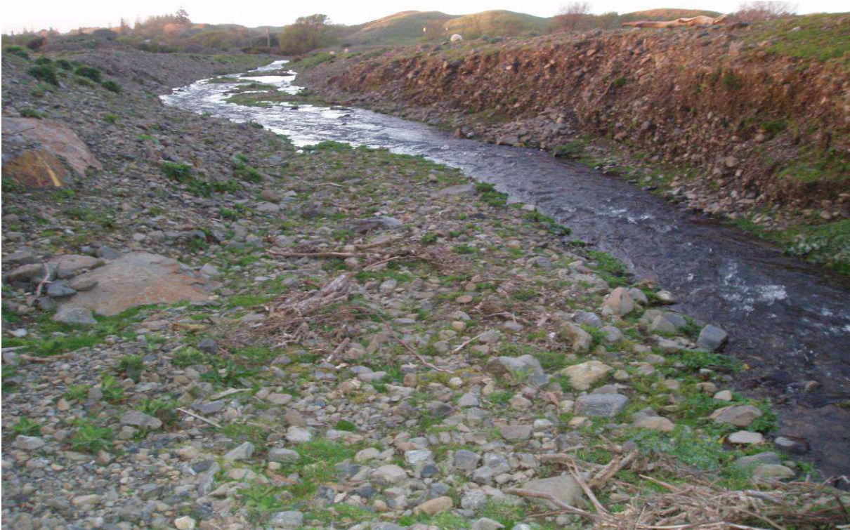
Figure A5 Smith Creek Site 3 just below the SH1 bridge
