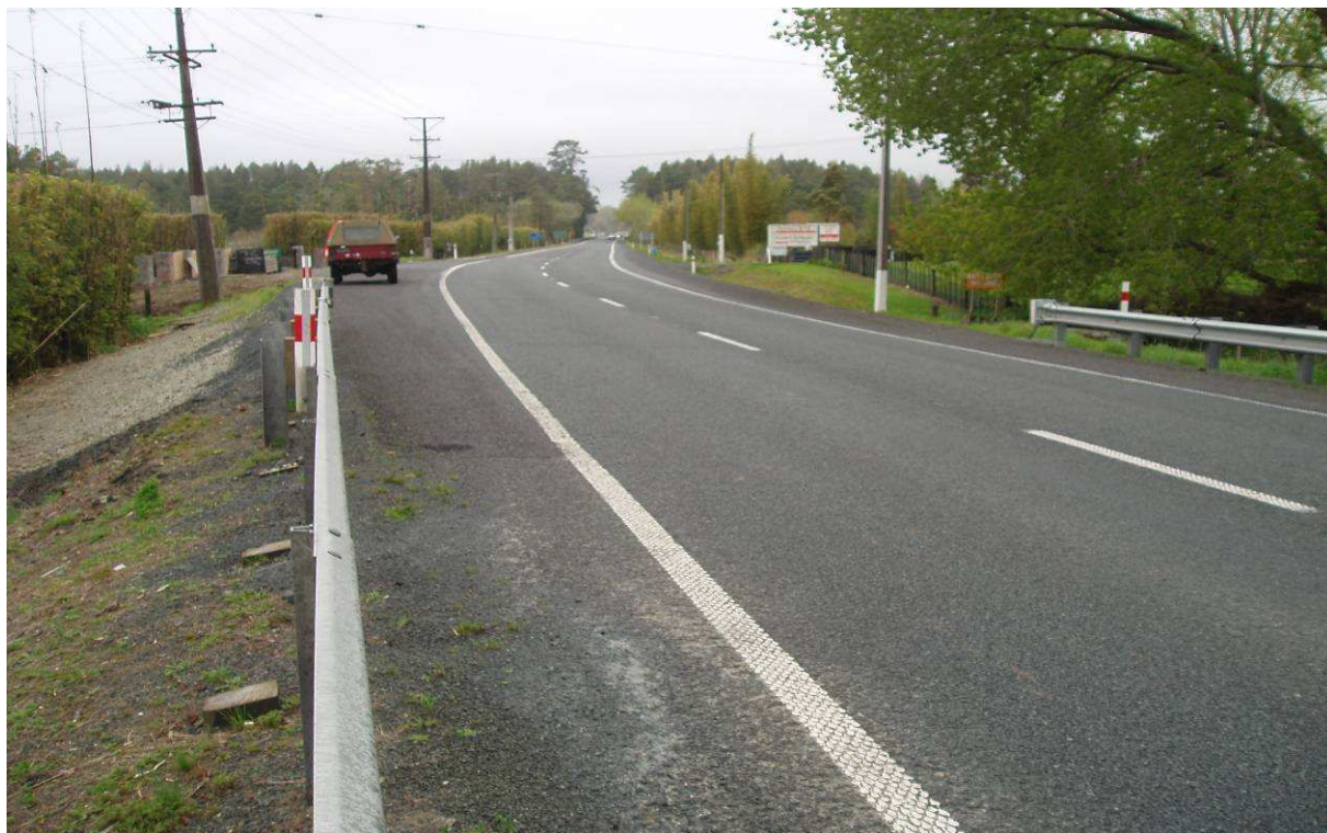
Figure A20 Roadside conditions at the North Branch of the Mahurangi River looking south towards Warkworth.
