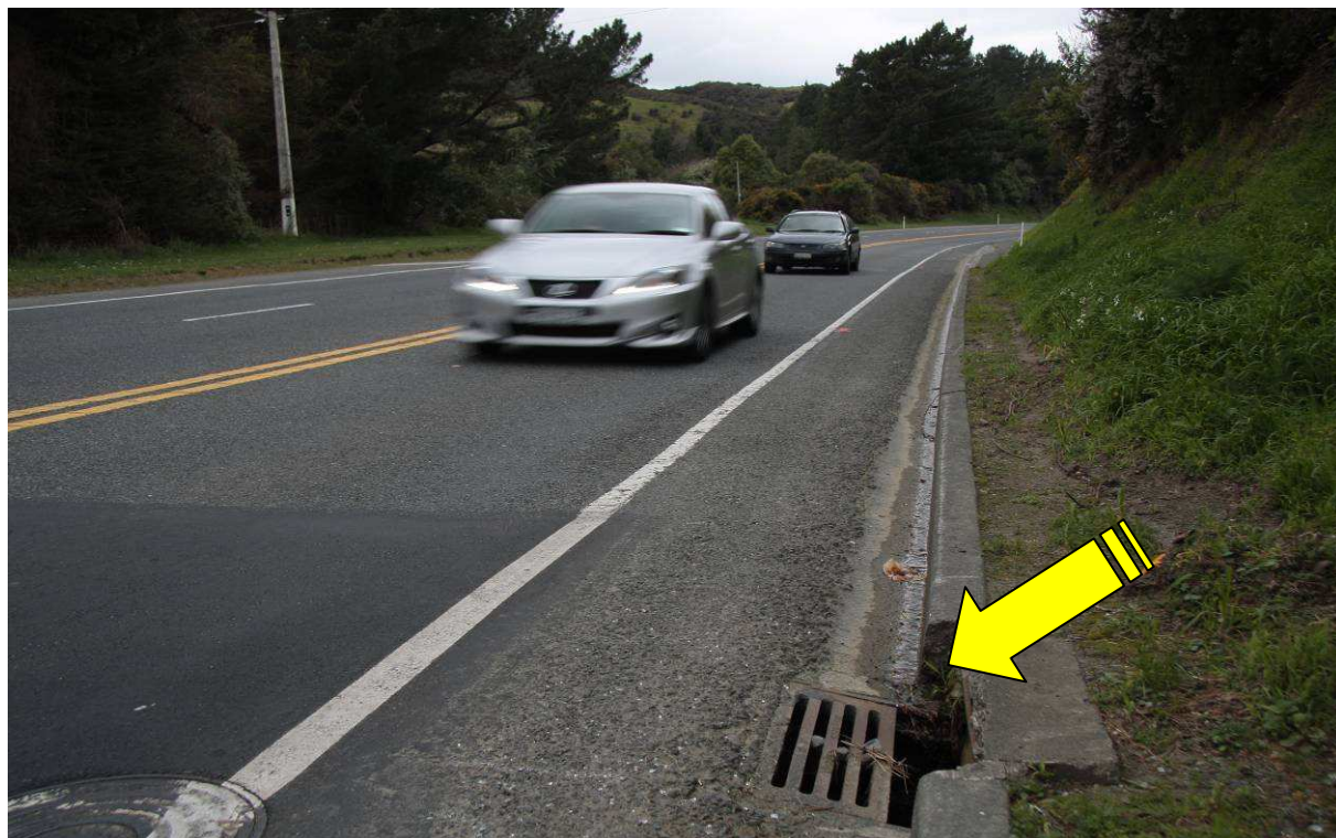
Figure A11 Roadside conditions at Pauatahanui Stream looking south at the base of a hill, showing the curb and channel and entry to the stormwater drain pipe that discharges on the stream (arrowed)
