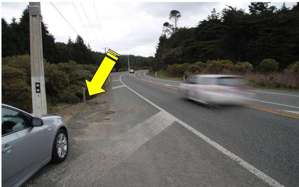
Figure A15 Roadside conditions at the small unnamed SH58 stream looking south towards a slight uphill bend in the road. The location of the stream below the road is shown (arrowed).
