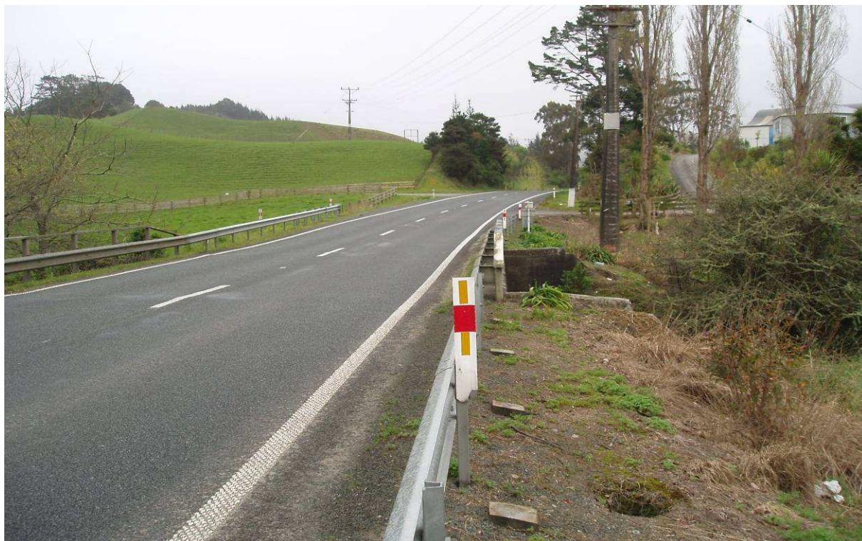
Figure A19 Roadside conditions at the North Branch of the Mahurangi River looking north towards a slight uphill bend in the road.
