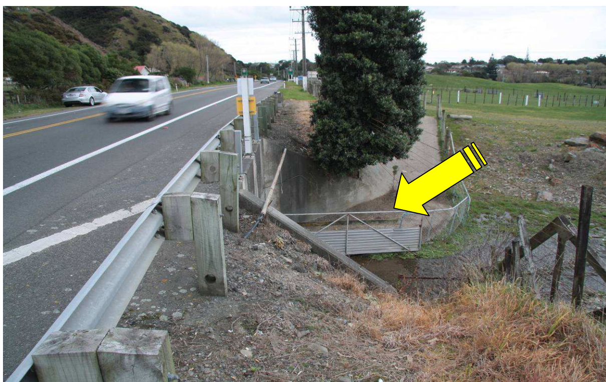
Figure A8 Smith Creek looking southward showing the sheep pass under SH1 (arrowed) that may have contributed localised sediment or nutrient inputs to change invertebrate communities slightly
