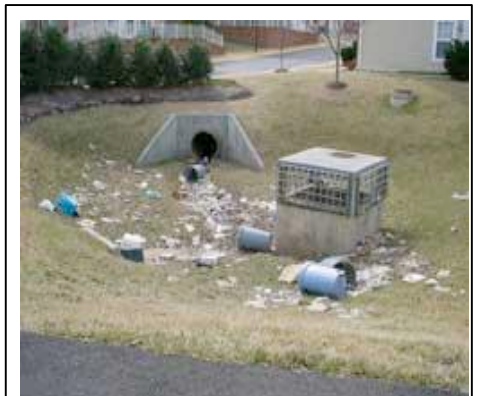
Deposited litter in a dry stormwater detention pond
