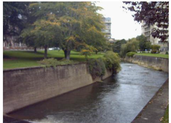
Lined section of the River Leith, Dunedin, 2005 Source: Otago Regional Council Leith Lindsay Flood Protection Plan (2005).
