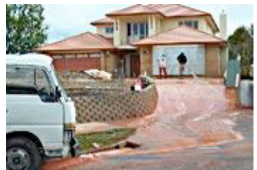
Building wastes spilling to road and stormwater system
